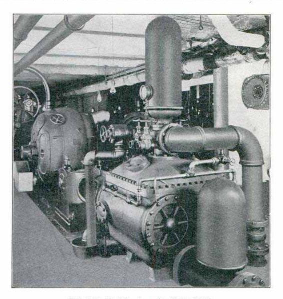
Electric Fire Protection Apparatus Always Ready.
