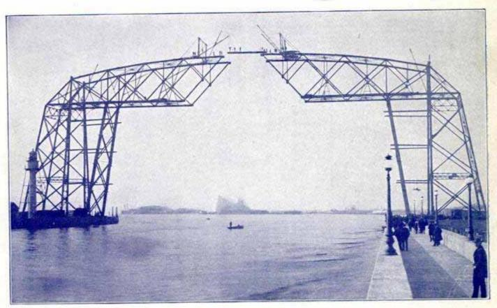
Placing the Steel Girder Which First Connects the Mighty Spans-The Workmen are 250 Feet above the Water-Only Structure of its Kindon this Continent-See Page 106.
