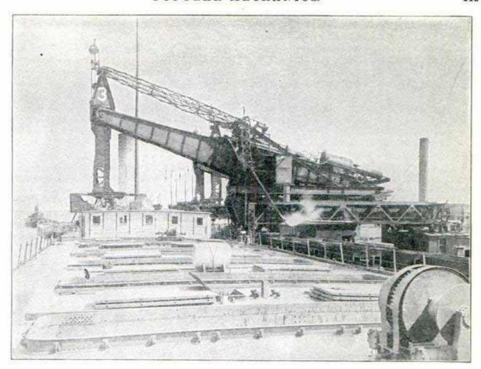
The Bucket Leg with Bucket Open and Ready to be Lowered into Vessel's Hold
