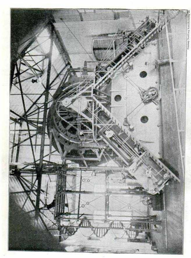
5,000 Horse-Power Hoisting Engine for Tamarack Mine-Weight 1,200,000 Lbs.
