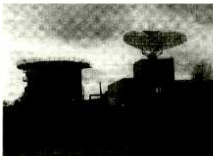
All that is supposedly left of Camp Hero in Montauk, NY is this remnant of a WWII Sage-radar system used for coastal defense. The terrain of Montauk Point is an extremely rocky bluff overlooking the Atlantic Ocean. Speculators rumor that a nearby bunker leads downward into a hollowed subterranean mountain. Could this be an eastern Mt. Cheyenne?
