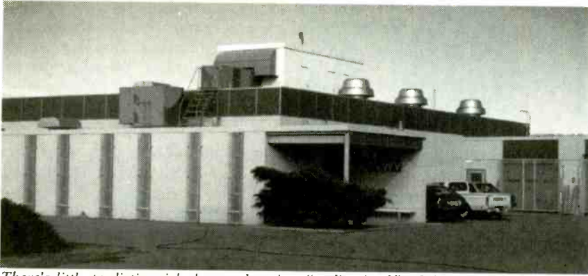
There's little to distinguish the nondescript "radio shack" of the NIST Radio Station WWV (located on East County Road 58 in Ft. Collins, CO), except for the station's familiar call sign, which is displayed prominently in the building's entranceway.
