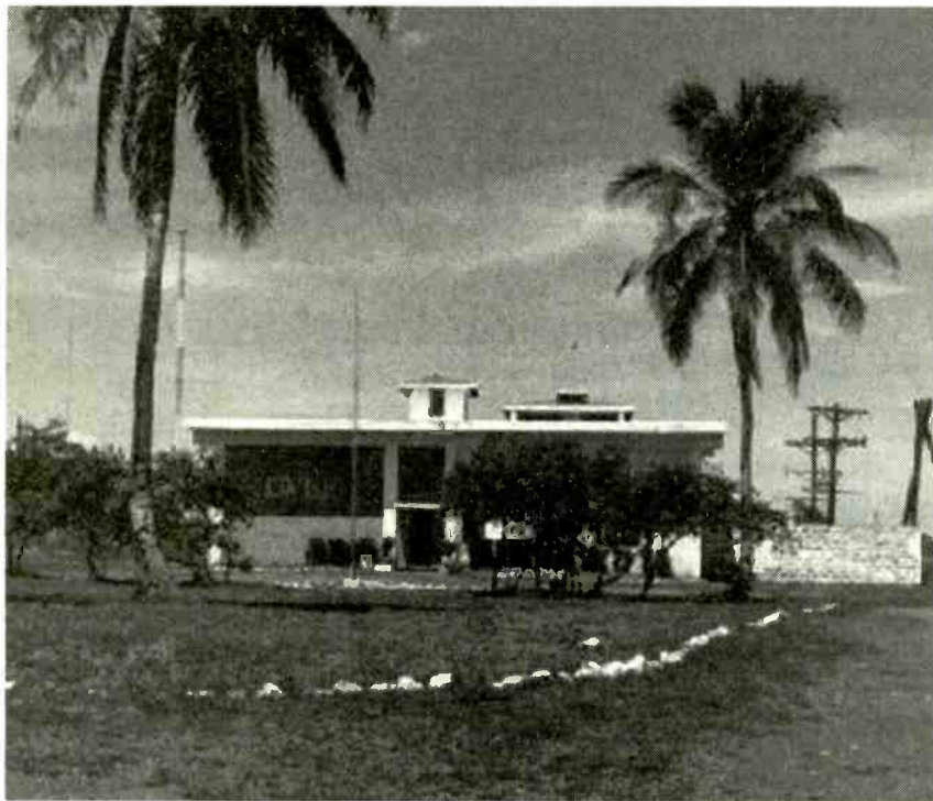
Here's a photo of the Far East Broadcasting Company's transmitter building at Iba, in the Philippine province of Zambales. If you'd like to check out other views of the station, visit FEBC's website at http://www.febc.org/febchom.html .
