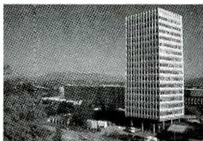
The International Telecommunication Union's modern headquarters building, shown here, is located in Geneva, Switzerland.
