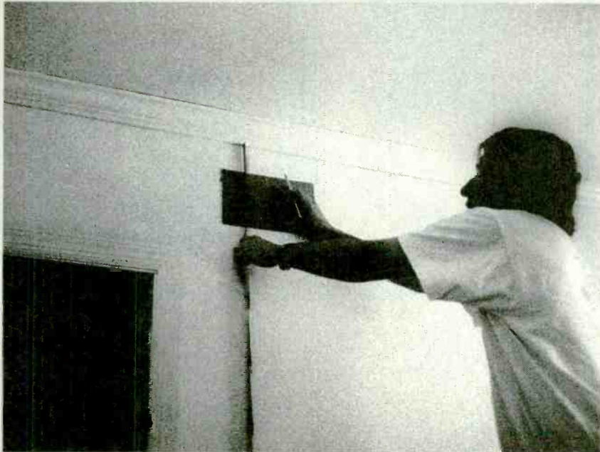
The template supplied with the speaker makes it easy to mark the locations for the holes to be cut.
