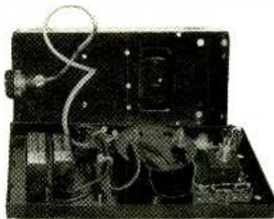
Most of the monitor circuit was assembled inside an electrical breaker box on a five-lug tie-point barrier strip, and connected to the meter, the power source, switch and LED's via hook up wire.
