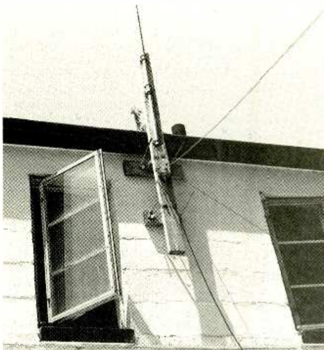
Here is what my antenna actually looked like. Six to eight lengths of 2 \times 4 were first mounted to the wall to provide a stable mounting surface for the antenna.
