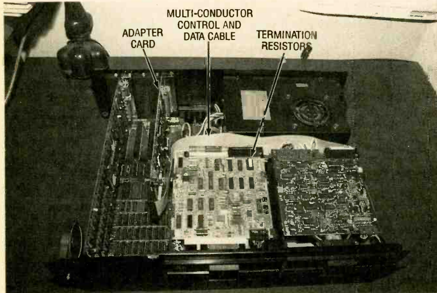
The actual position of the cable connectors may vary from one PC to another, but they are easy to identify if you take note of where they terminate.
