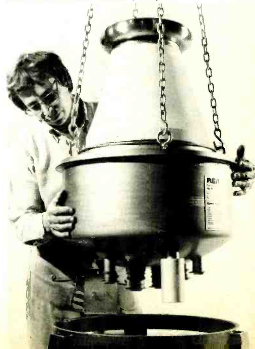
Fig. 2. The largest (320 lb) water-cooled tube of its kind ever made. (RCA)
