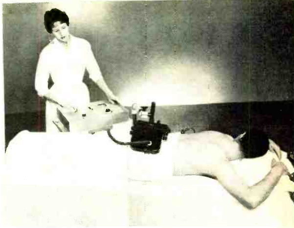
Diathermy machine, made by Burdick, operates on frequency of 27.120 MHz.
