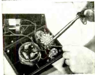
Construction of Multimeter.
