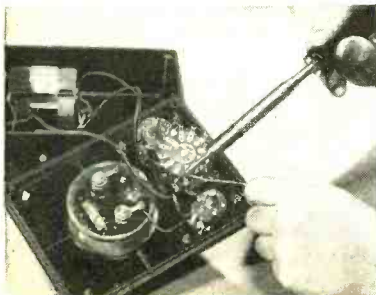
Construction of Multimeter.
