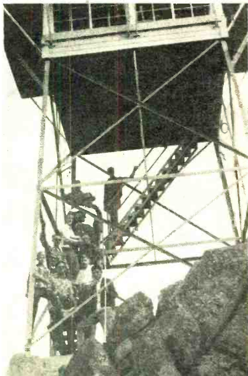
Members of Prescott (Ariz.) Emergency Radio Association (REACT) line up on a fire lookout tower operated by the U.S. Forest Service. In cooperation with the Forest Rangers, they have installed a base station in the tower on 7700-ft. Spruce Mt.
