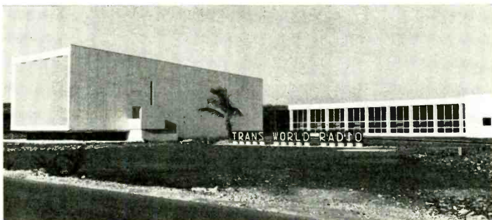
The new studio and office building of Trans World Radio , Bonaire, Netherlands Antilles, is one of the most advanced of its type in the world. It is unique in that it has acoustical floating walls, reverberation control, absorption panels and sound proofing. The gigantic antenna complex was erected several years ago.
