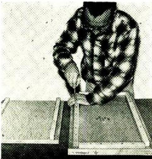
Fig. 2. Start assembly by joining cleats to bottom (left) and cleats and glue blocks to side (right).
