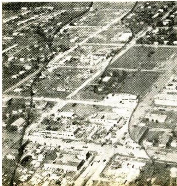
The tornado that swept through Hale Center, Texas, last June, demolished three farm homes (including that of Floyd Shackelford, below, right), left five dead, and hundreds homeless. The CB'ers in the area risked their lives to warn and protect others.
