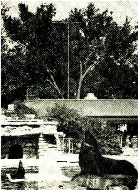
The building in the background is the main control center for 13 base stations located throughout the St. Louis (Missouri) Zoo. The sea lion in the foreground appears to be imitating the antenna, a Mosley "Devant-1," perched on the roof of the building.
