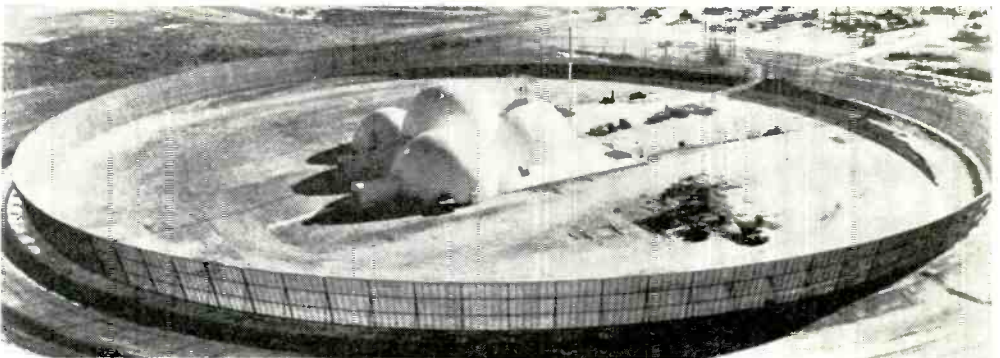
ANTI-MISSILE RADAR —Experimental radar system developed by Sylvania employs many antenna elements rather than a rotating dish to track enemy missiles. The radar beam is steered electronically by shifting electrical phase of individual elements.
