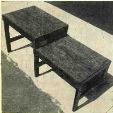
The work/op bench in various stages of assembly. Use screws and shun glue, and you can easily take it apart for moving, set it up later on.
