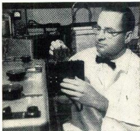
Dr. John B. Henry operates an electronic enzyme analyzer; the enzymes found in blood and other body fluids are essential to good cell functioning.
