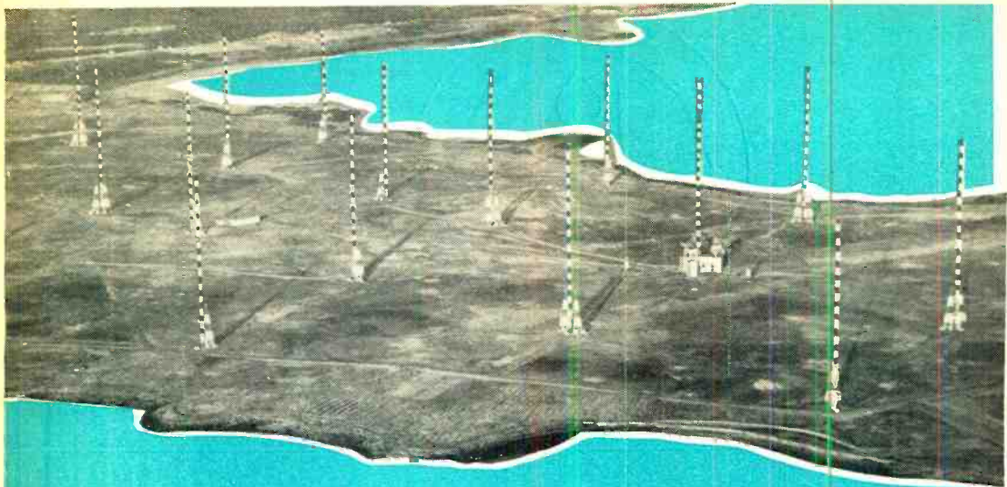
Antenna system at NAA, the Navy's Cutler, Maine, VLF radio station, covers two square miles, and consists of two arrays, each resembling a six-pointed star. The antenna system is actually a network of cables supported at an average height of 600 feet by 26 towers ranging in height from 800 to 1000 feet. In effect, the antenna is one plate of a huge capacitor—the elaborate ground system is the other plate—which couples NAA's tremendous output power to the atmosphere. Huge antenna and high power allow communication with submerged submarines.
