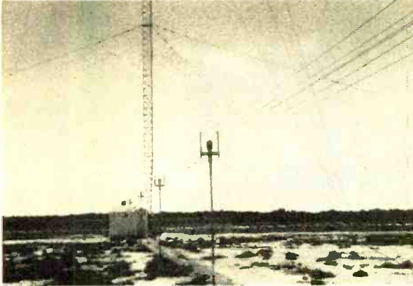
Three towers (one is shown above with its transmission line) are used in the highly directional Radio Marathon antenna array. Signal in U.S. is weak.
