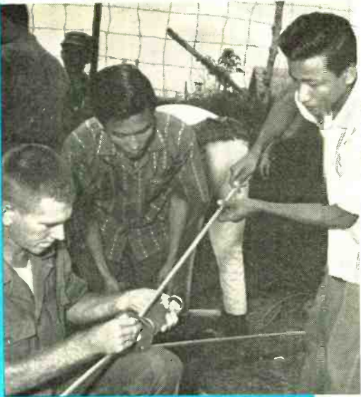
Both USOM technicians and South Vietnamese troops helped local villagers install antennas for their nation's "40-megacycle intercom." Flag near antenna in bottom photo is South Vietnam's national banner; it consists of three narrow red stripes in a yellow field.
