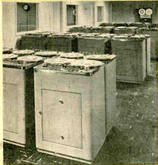
Discs are then transferred to tape on one of the 32 machines in the Muzak recording studios (left). Tapes are played back (right) on equipment at local franchised distributors.
