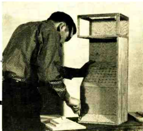
Side view of enclosure, showing its perforated resistive panel. All joints are screwed and glued.
