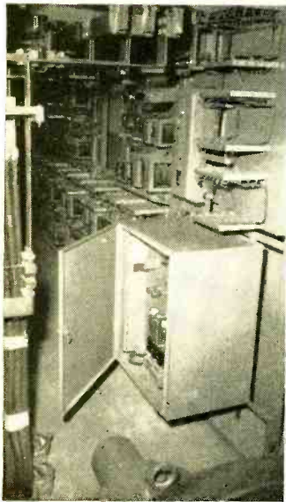
Thanks to magnetic amplifiers, this paper-making machine at West Tacoma Newsprint Corporation in Tacoma, Washington, can operate at 5000 feet per second, many times faster than previously possible. Magnetics continuously adjust the speed of the take-up rollers, slowing them down as the roll of paper gets larger. Control room is at left.
