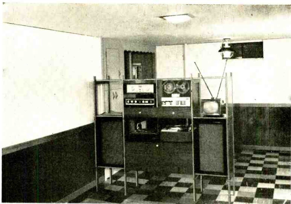
Treatment of test room with acoustical tile results in better room acoustics and better looks, too.
