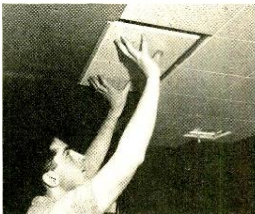
Enjoyment of hi-fi —especially stereo—can usually be improved by installing acoustical tile in the listening area.
