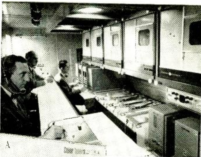
Mobile unit houses complete Eidophor system. At right is view of control room in the 35'-long motor trailer.
