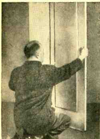
With Fiberglas in place, attach the panel.
