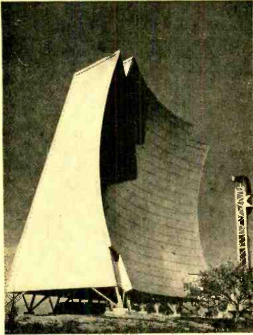
Giant over-the-horizon antenna designed by Bell Telephone Laboratories for "White Alice," Air Force Alaskan defense communications network.
