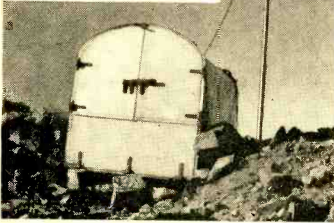
Translator is housed in small weatherproof shack (below). Note antenna at right. Programs are beamed out on one of the u.h.f. channels. Programs that originate on a u.h.f. channel may also be "translated" with a frequency converter and then retransmitted.
