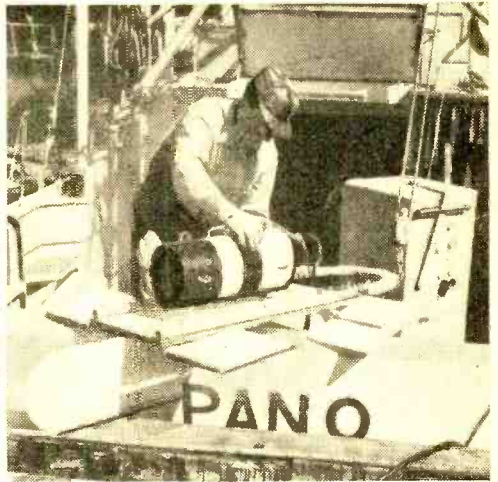
Underwater TV housing being mounted on sled (above) prior to use at Coral Gables, Fla. The camera within the housing scrutinizes fishing gear while it is in operation.
