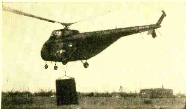
Complete microwave station dangles from this Air Force "egg beater" to be taken to hard-to-reach location. Within two hours after arrival, station will be sending radar data over six radio frequencies that may be split into 24 telemetering or 72 two-way voice channels. (Photo courtesy Motorola, Inc.)
