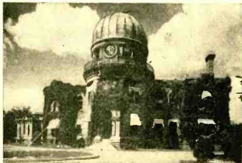
The Dominion Observatory, Ottawa, Ontario, Canada, is surmounted by a dome which houses a 15-inch equatorial telescope. The Positional Astronomy Division, of which the time service described in the text is a part, has its transit instruments housed in the left wing.
