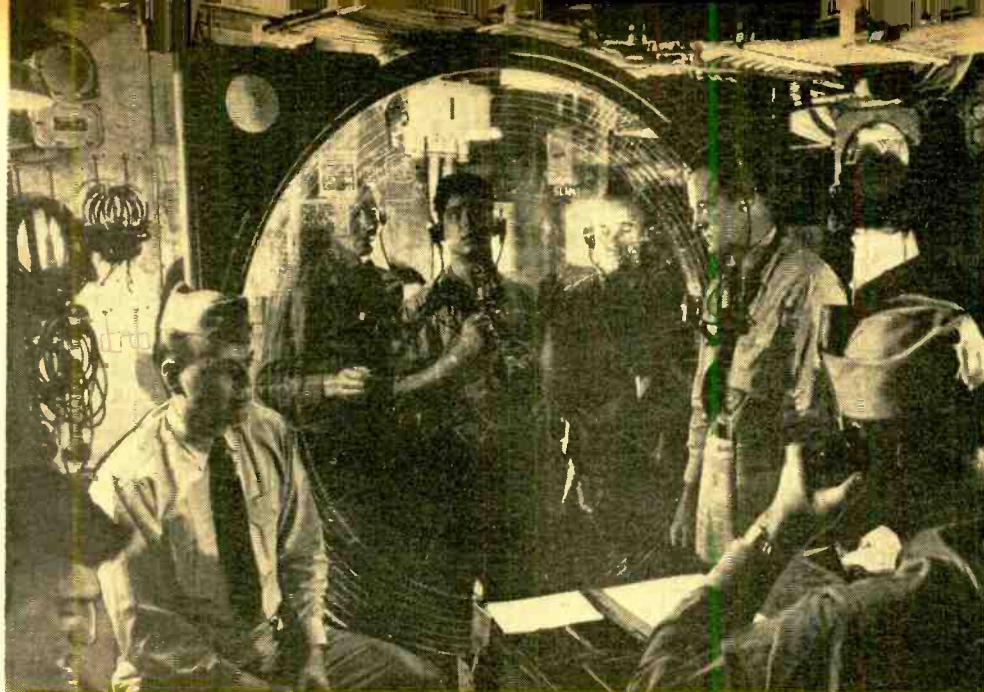
Data gathered by radar operators, picket ships, radio contacts, etc., are displayed on vertical plotting board which reveals an up-to-date picture of air activity.
