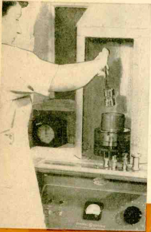
A General Electric ultrasonic generator is shown being used at the Holley Carburetor Co. to clean a jet engine fuel control part.
