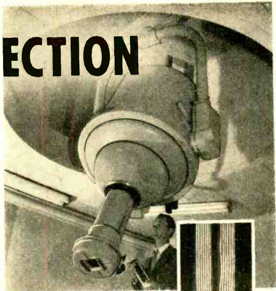
Anode of this gigantic x-ray unit gets one million volts. G-E built it for Sutter Hospital, Sacramento, California.
