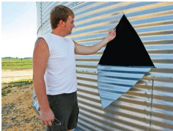
Baker shows a gash cut into the silo to release grain.
