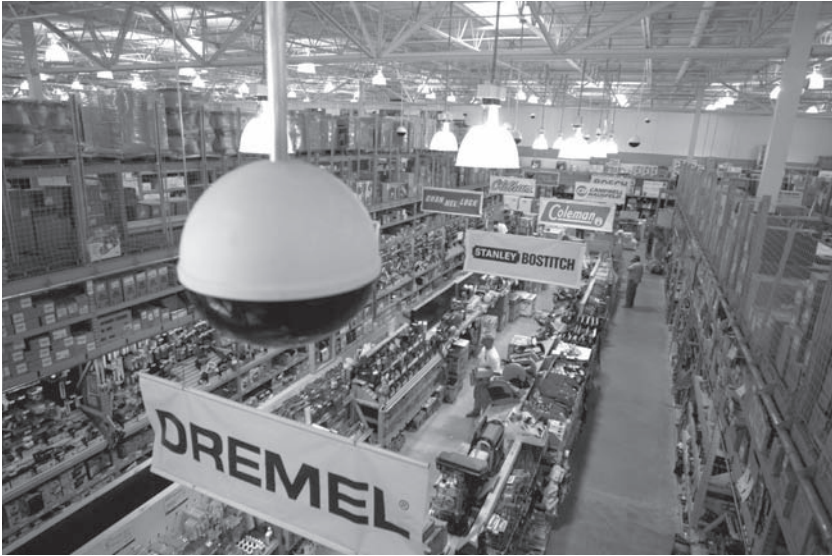
Figure 9-1 Dome Camera In Retail Facility
