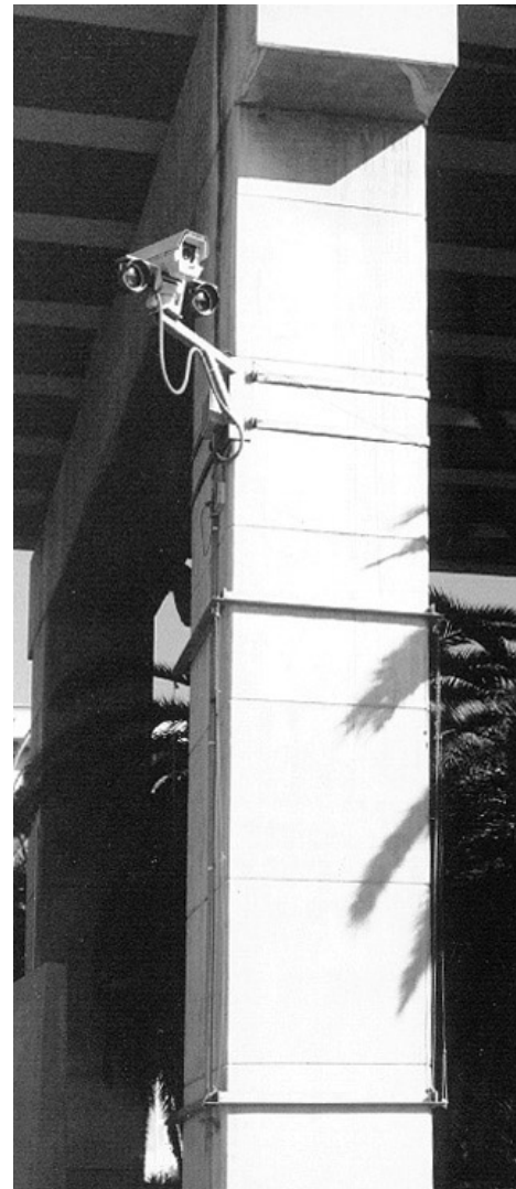
Strapping a bracket around a concrete column
