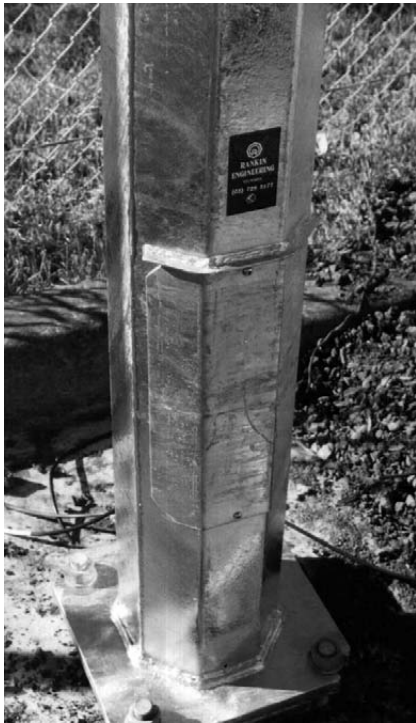
A hexagonal metal pole is stiffer than a circular pole
