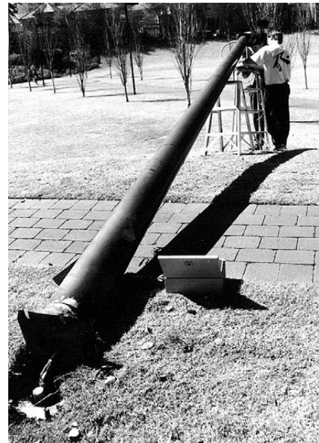
Hinged PTZ camera pole makes servicing easier.
