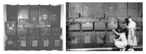
Left: The ENIAC computer, constructed in 1945 and rolled out in February 1946, was essentially a giant advanced calculator which was used for a variety of U.S. Army projects including ballistics calculations, scientific computing, weather prediction, and thermal ignition studies. Right: Programmers are shown changing the coding configuration by physically rearranging the wires. [U.S. Army historical photos, public domain.]
