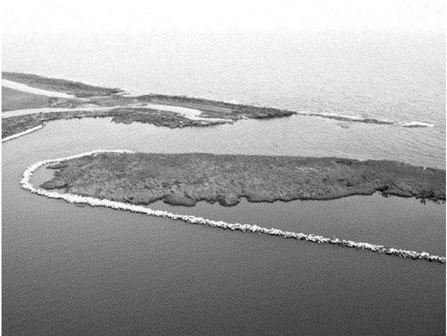
Top Left: Colonel Crear arriving for the Mississippi Delta Wildlife and Wetland Tour in the Vicksburg District in 1987. Top Right: Alligator mom in the Mississippi wetlands, just one of the many species observed during the Wetland Tour. Bottom: Erosion protection measures are illustrated where the mouth of the Mississippi River flows into the Gulf of Mexico, including banks and rock dikes, 1994. [U.S. Army Corps of Engineers news photos, released.]
