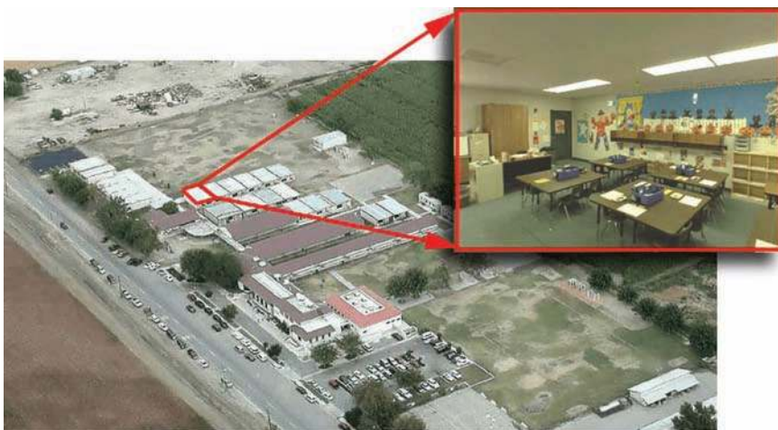
Figure 6.35 PANOSCAN PHOTO SEQUENCE VIRTUAL MAPPING. The images in this sequence were converted to an interactive QuickTime VR presentation, which allows the user, by simply rolling the mouse cursor over any room, to make a virtual “leap” into that room. (Courtesy of Mr. Casey Coss, C.F.O., Panoscan, Inc., www.panoscan.com .)
