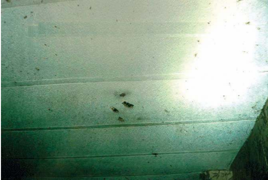
Figure 22.4 CEILING IN VICTIM'S BEDROOM. Ceiling in the victim's bedroom directly above the body. If this event had transpired as presented, the ceiling would be splattered with blood and brain matter. Furthermore, if you look closely, those defects in the ceiling are actually from a muzzle blast, as if someone had pointed the gun towards the ceiling and fired off two rounds. (From the author's files.)
