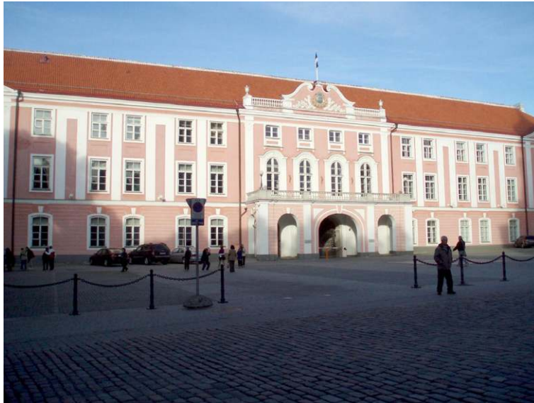
FIGURE 2.2 Toompea Castle in the upper town of Tallinn is the home of the Estonian Parliament. A Denial of Service attack in April 2007 caused the Parliament’s e-mail servers to become unavailable, delaying the Estonian government’s response to countrywide cyber attacks at the time. Source: CIA World Fact Book.
