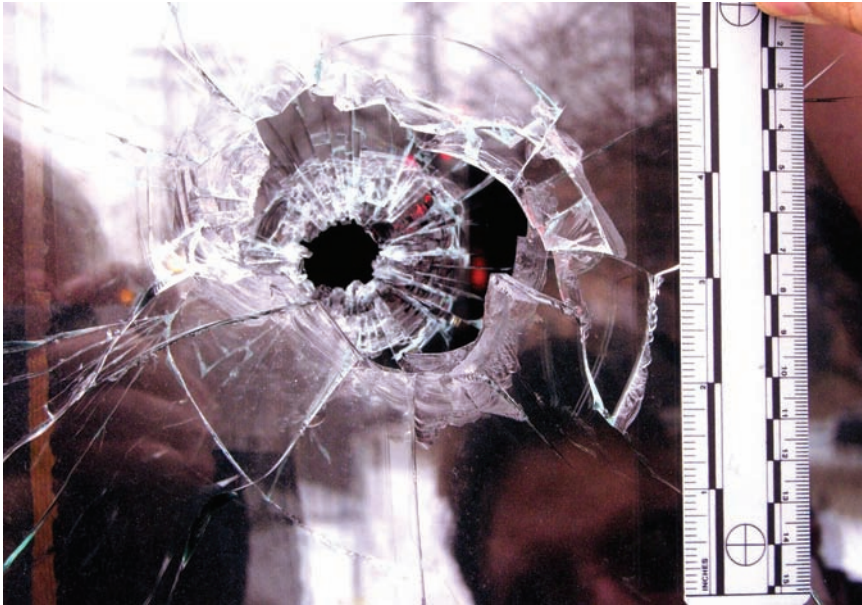
Figure 17.40 OUTER WINDOW — SHOTS FIRED THROUGH GLASS. The outer window has an irregularly shaped hole caused by the bullet beginning to tumble after exiting the inside window — proof that shots were fired from inside the club and out toward the plate glass door. (Courtesy of Detective Mark Czworniak, Chicago Police Department.)
