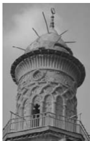
The minaret of the hospital, madrasa, and mausoleum of Sultan al-Mansur Qala'un, built in the 13th century, still bears the protruding wooden rods at its peak from which Ramadan lanterns were once hung.
