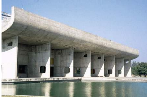
Fig. 12.2 Le Corbusier's Assembly Hall in Chandigarh borders a water tank and makes direct reference to local palace architecture that overlooks picturesque lakes
