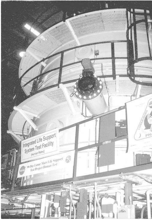
Figure 42.4 Twenty-foot circular building.
