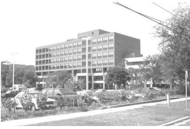
Figure 28.6 Vegetation blocks views to this health facility's main parking structure and its entrance.
