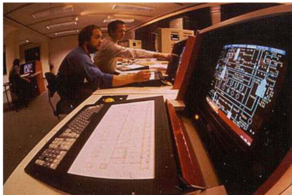
Fig. 8.3 Mixed instrumentation refurbishment of a 1970s power plant
