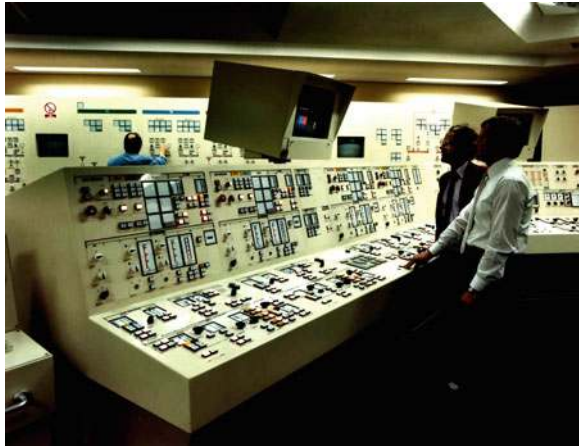
Fig. 8.2 The CEGB modular instrumentation as implemented at Heysham 2
