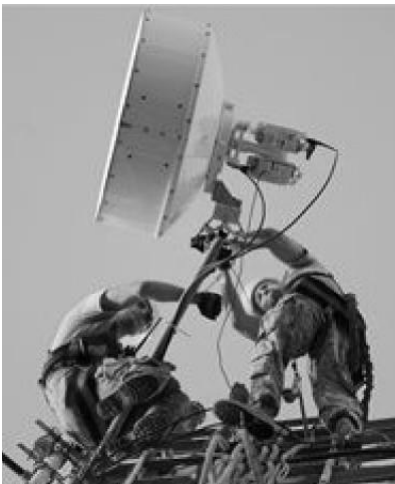
Left: U.S. Air Force crew adjust a microwave communications antenna atop a communications tower to provide wireless network access. Right: This transceiving dish was installed in Kandahar, Afghanistan, to provide wireless in-the-field telephone and Internet communications via orbiting satellites. [News photo by Staff Sgt. Mike Meares and Sgt. James Harper courtesy of the U.S. Air Force, 2011 and 2009, released.]
